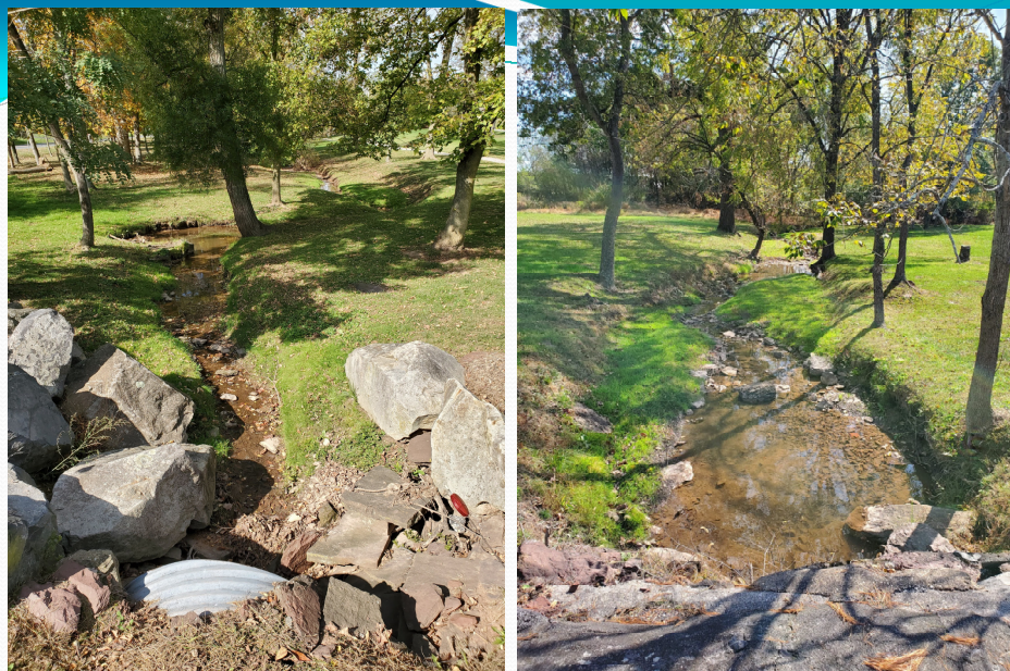
Stream Restoration at Adams County Human Services
