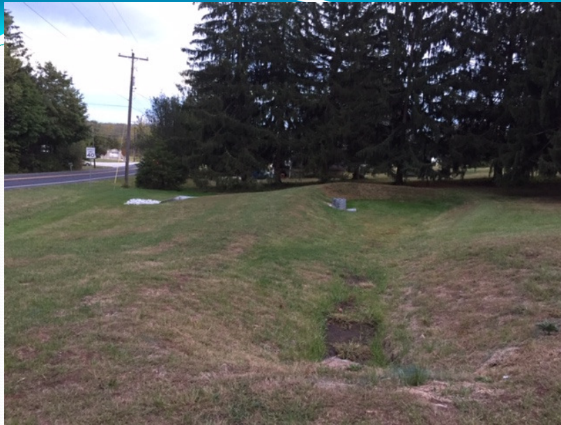
Longview Blvd East Basin
